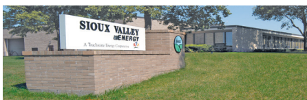
Sioux Valley Energy's headquarters, Colman, S.D.
